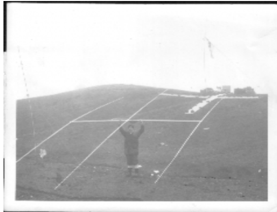
The 20M beam ready to go up. The cross on the hillock behind is a survey marker. The 36ft vertical is sited here too.
